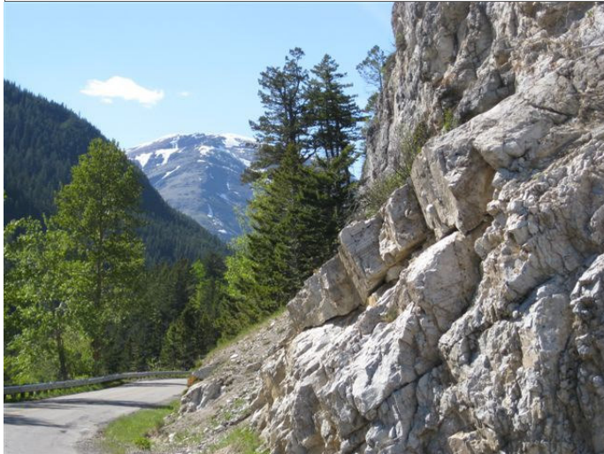
Reference Photograph: This scene depicts the curvy road going up to Red Rock Canyon in Waterton Lake National Park, Alberta.
